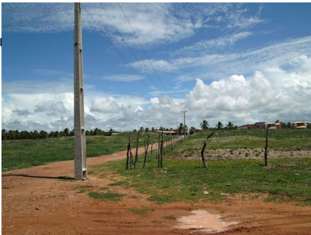
The new electricity pylons with power going into PDC
